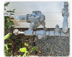
PHOTO — GAS UTILITY
