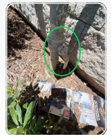
PHOTO — MAIN SHUTOFF LOCATION
